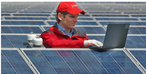
Figure 2 Two SR30 secondary standard pyranometers measuring GHI (global horizontal irradiance) and POA (Plane of Array) in a PV performance monitoring system
