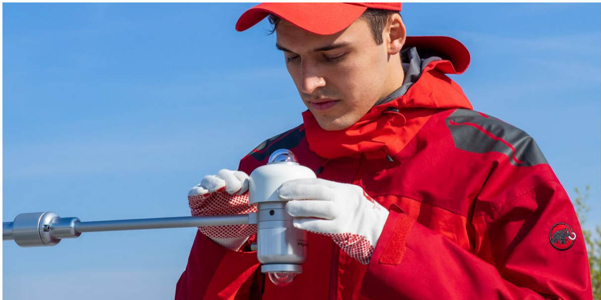
Figure 0.4 Installation with AMF03, two SR30-D1 pyranometers, and ALF01 levelling fixture
