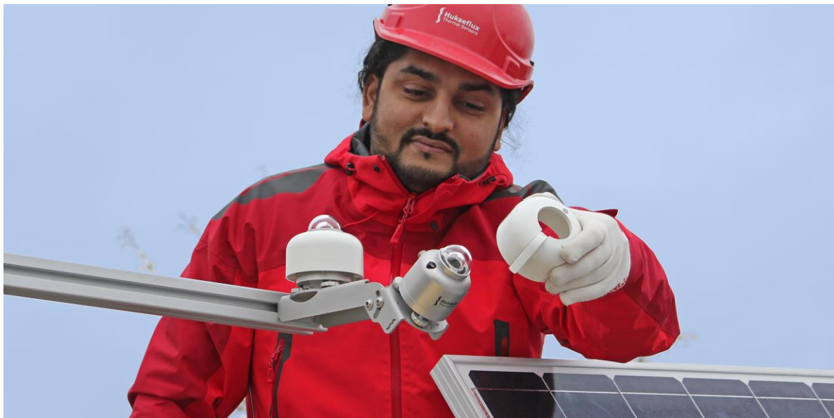
Figure 0.6 PMF02 is uniquely designed for PV system performance monitoring with two pyranometers, one in Plane of Array
